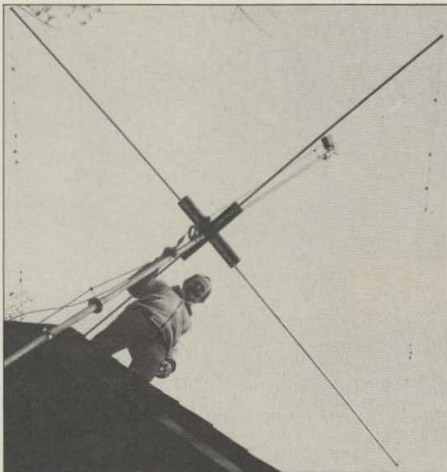
Photo A. The completed X-beam.
